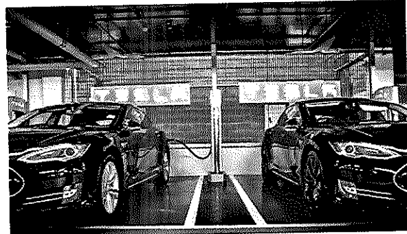
Supercharger station, indoor
