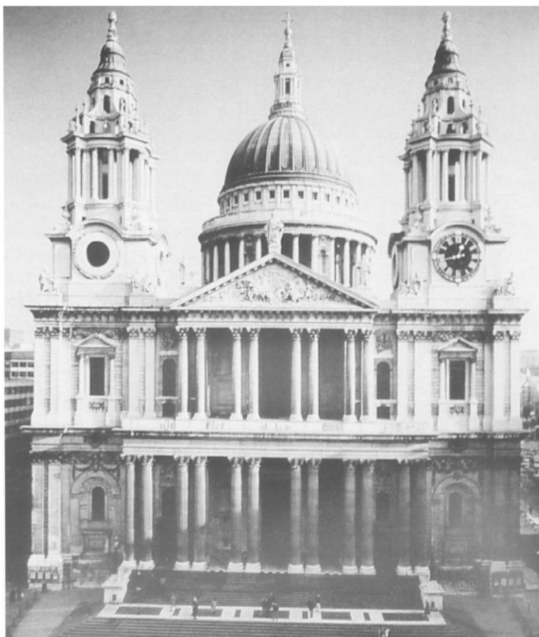
Figure 1. St Paul's Cathedral. (© Guildhall Library, Corporation of London.)
