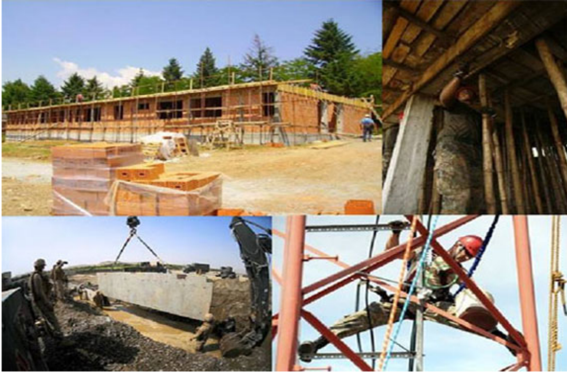
United States Army Corps of Engineers construct a community center in Varvarin, Serbia; a Marine electrician removes wood used to form a concrete ceiling in Bangladesh; Navy Seabees place concrete pieces at the Musa Qal'eh project in Afghanistan; An Airman balances on a communications tower in Westhampton Beach, New York.
