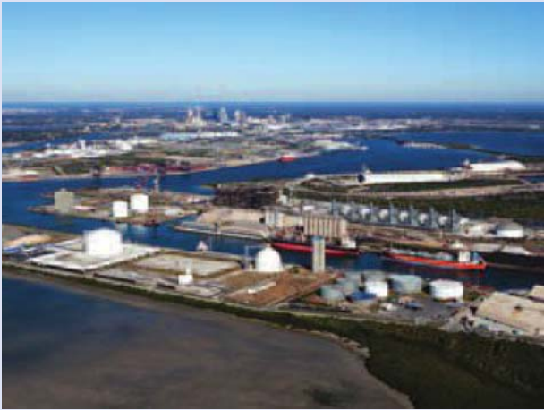
Bulk terminals in Tampa, Florida are some of Kinder Morgan's above-ground tangible resources.
