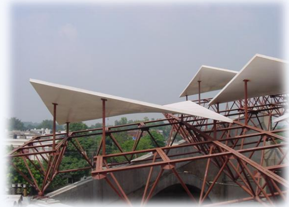
SPACE FRAME STRUCTURE
