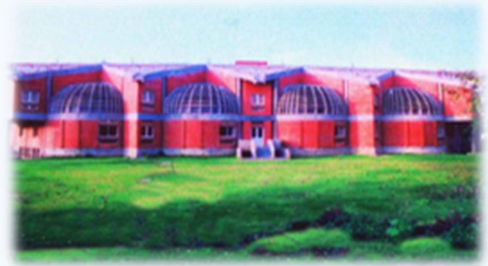
SOUTHERN VIEW OF PEDA OFFICE COMPLEX
