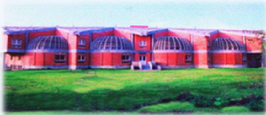
SOUTHERN VIEW OF PEDA OFFICE COMPLEX
