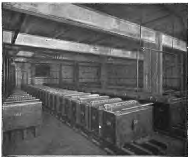
Fig. 115. E.P.S. Storage Battery
