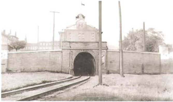
Figure 6.12 The Brockville Tunnel, Canada's first railway tunnel, took more than six years to construct.
