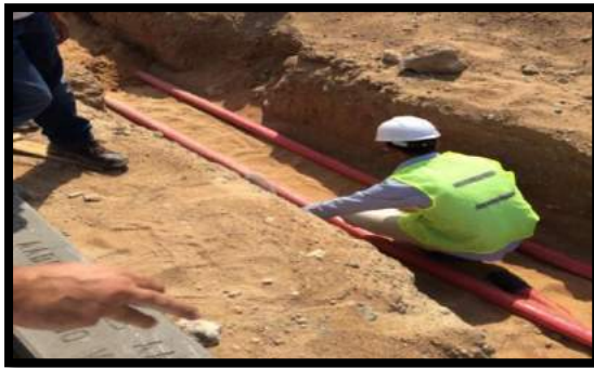
Fig 2.1.8 Distance between 11KV cables
