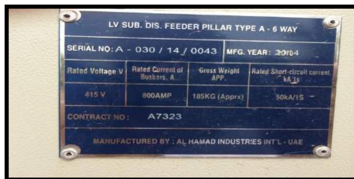
Figure 2.2.1 serial number of Transformer
