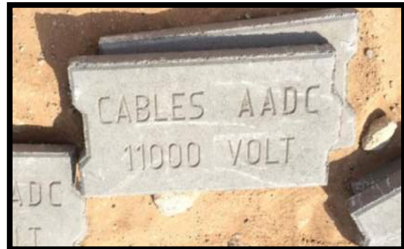
Fig 2.1.9 Cement Pieces to protect cable
