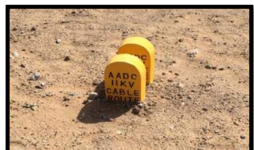
Fig 2.1.11 Warning fixed cement piece
