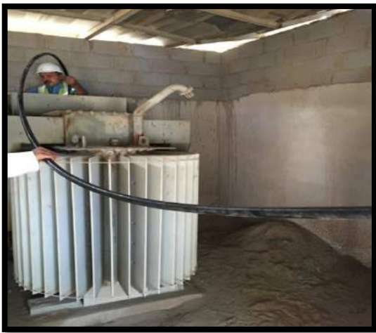
Fig 2.3.15 Filling the Transformer
